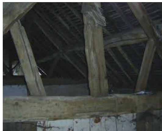
Fig. 4: Reused timber in barn roof truss
