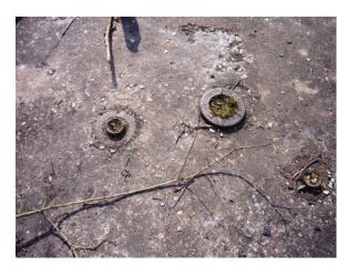
At the centre of each the position of the gun is marked by metal sockets in the ground to house the holdfast bolts that secured it in place. Each placement would probably have housed a standard 3.7 inch AA gun and the holdfasts were built to a standard pattern so that guns could be moved from site to site according to need.
